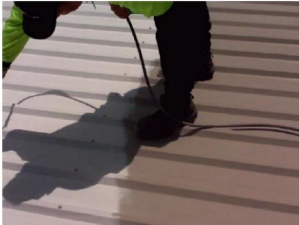
INSULATION MEASUREMENTS - WAREHOUSE ROOF
